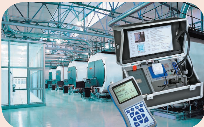
J2KN at Viessmann large boiler
